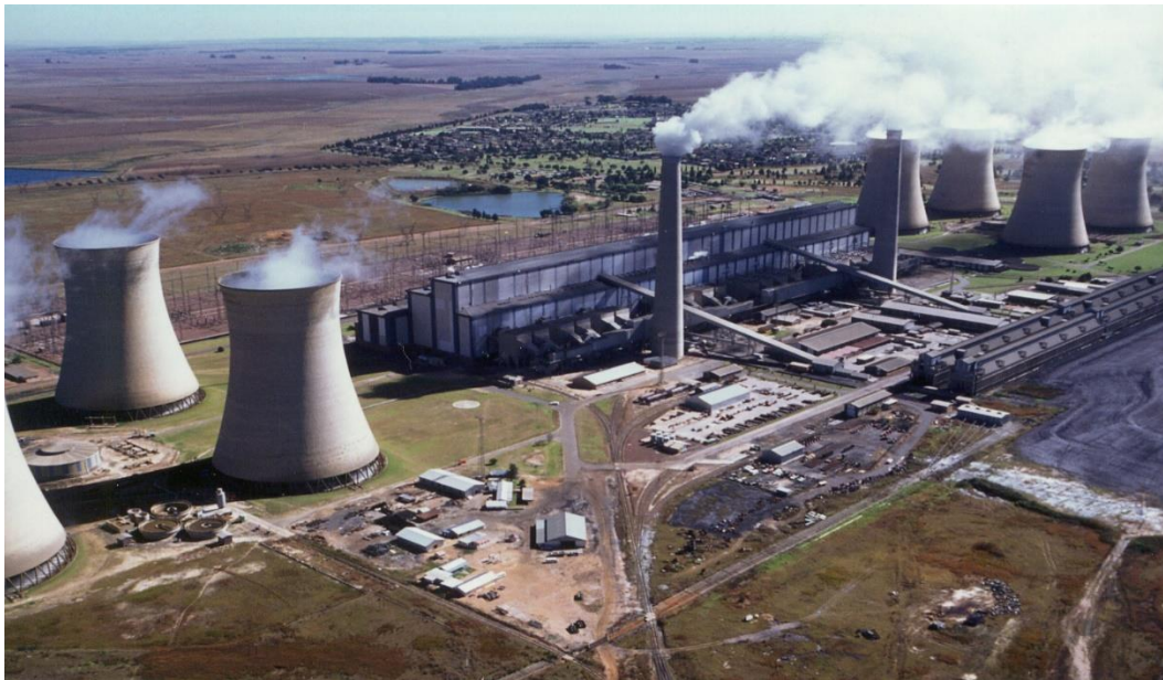
Figure 2.5: Hendrina Power Station in Mpumalanga, South Africa (Eskom)
