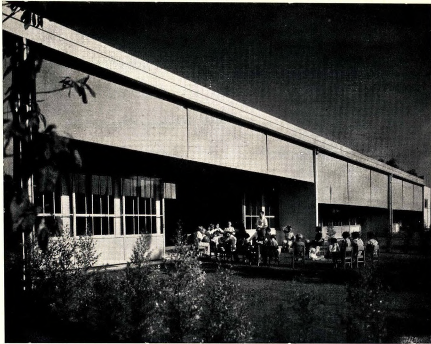
Indoor-Outdoor Classroom. Sliding glass front—mechanically operated awning
