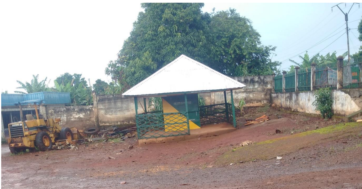
Figure 7-3: UCCAO's crumbling infrastructure.
