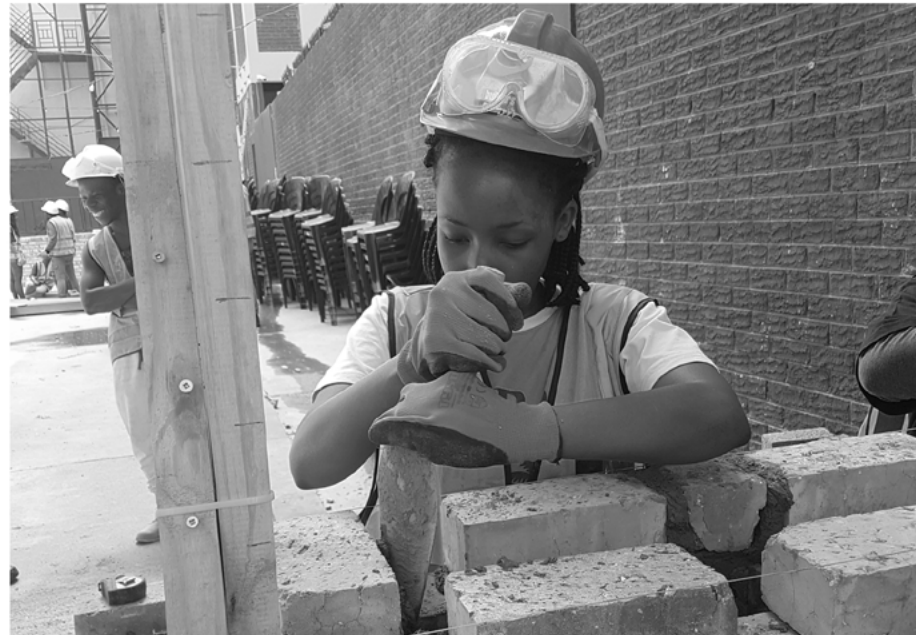
Figure 51: Jennifer Sibanda laying bricks at 94 Juta Republic in Johannesburg; photograph (Nevhutanda, 2017)
