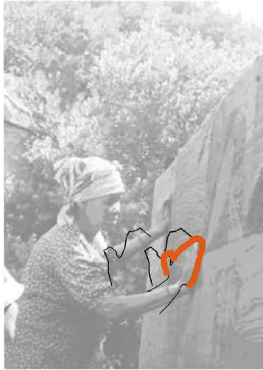
Figure 79: Actor making women - Using full face of hands as a light weight trowel; image source (Kammeyer, 2010); analysis (Nevhutanda, 2020)
