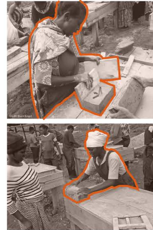
Figure 152: Local women of Rwanda brick making and shaping; photograph (Bruce Engel, not dated); source (Architizer, 2020)
