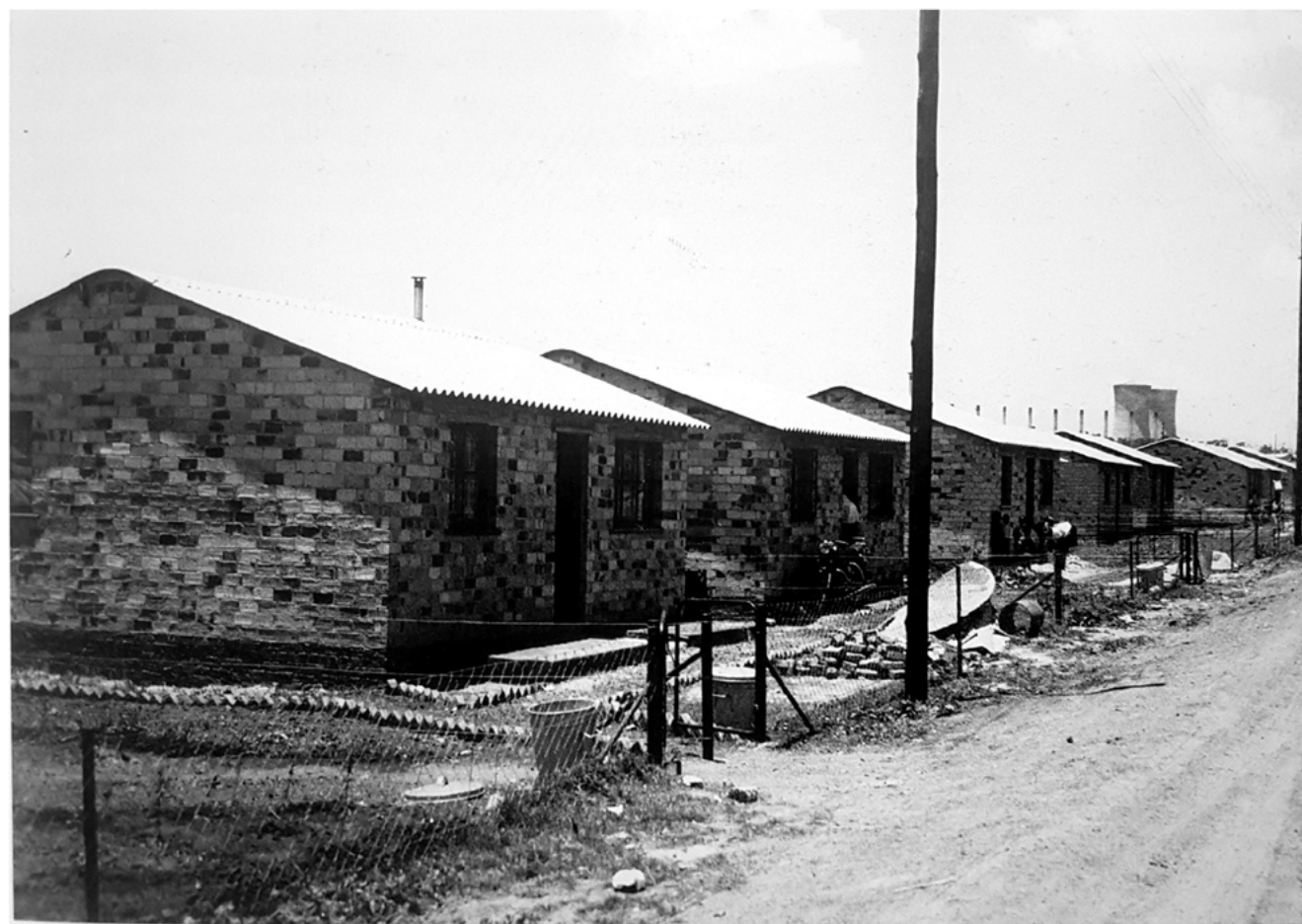
Figure 100: Housing built in Orlando in 1931; source (Wits historical papers from Nieftagodien, N & Gaule, S. 2012)
