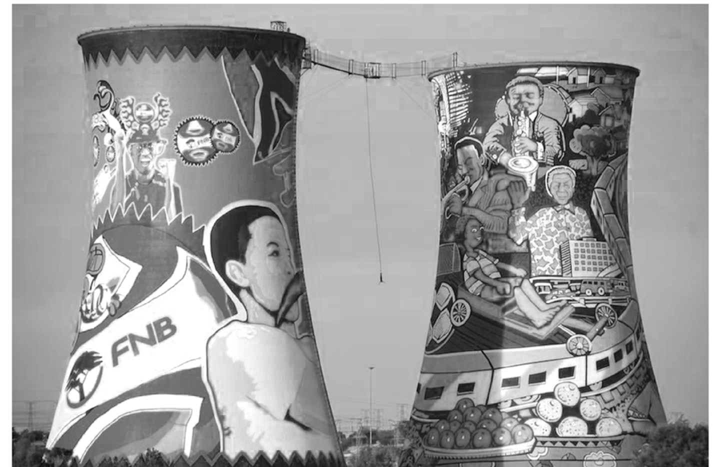
Figure 112: The Orlando Towers; source (Soweto Tours, 2020)
