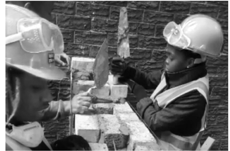
Figure 52: Researcher laying bricks at 94 Juta Republic in Johannesburg with her classmates; photograph (Jennifer Sibanda, 2017)
