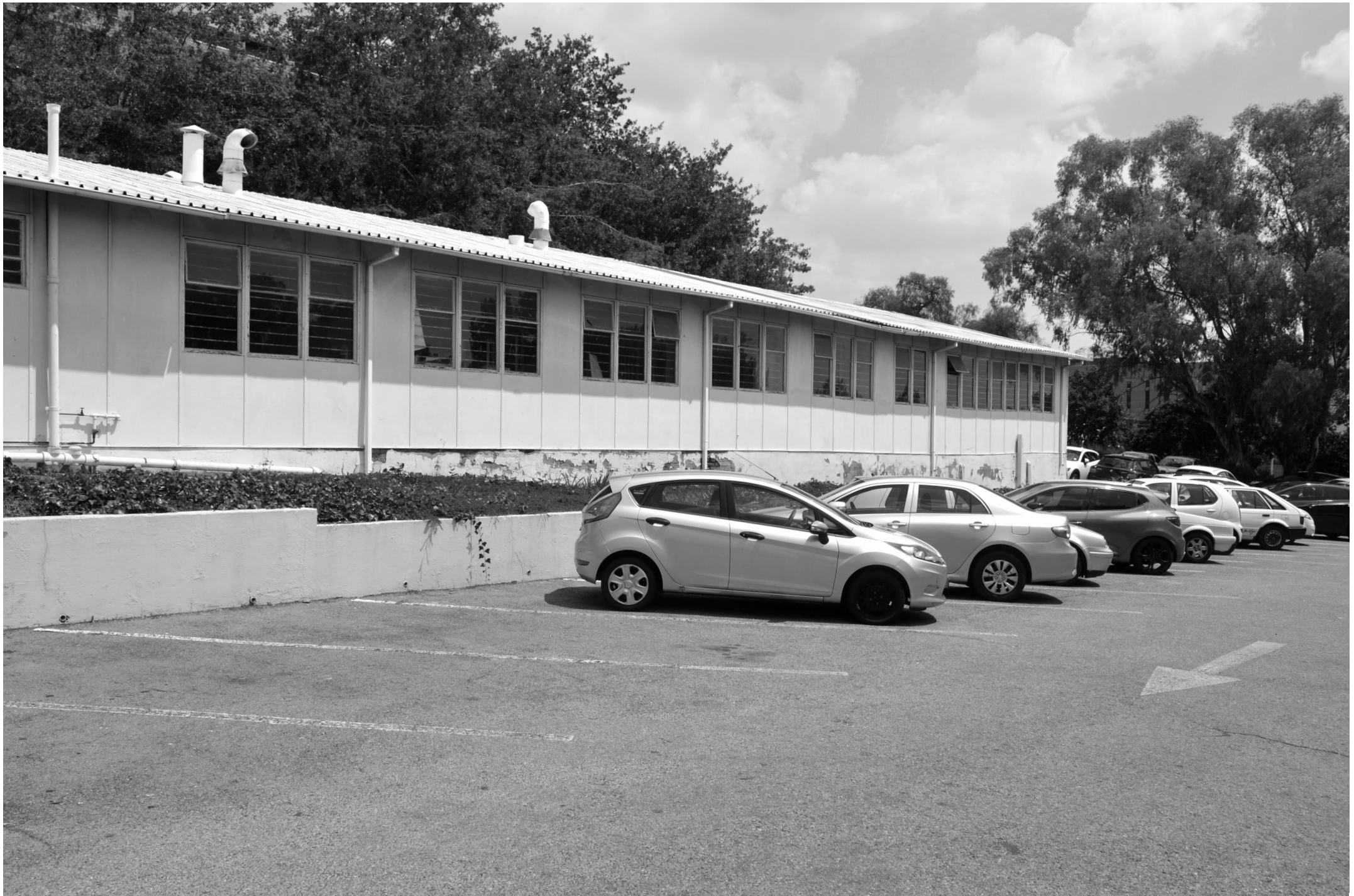
Figure 12. Photograph of the selected site showing the old architecture workshop looking south west.
