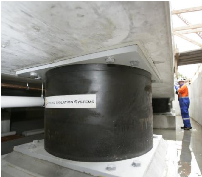
Figure 16. A base isolation system.
