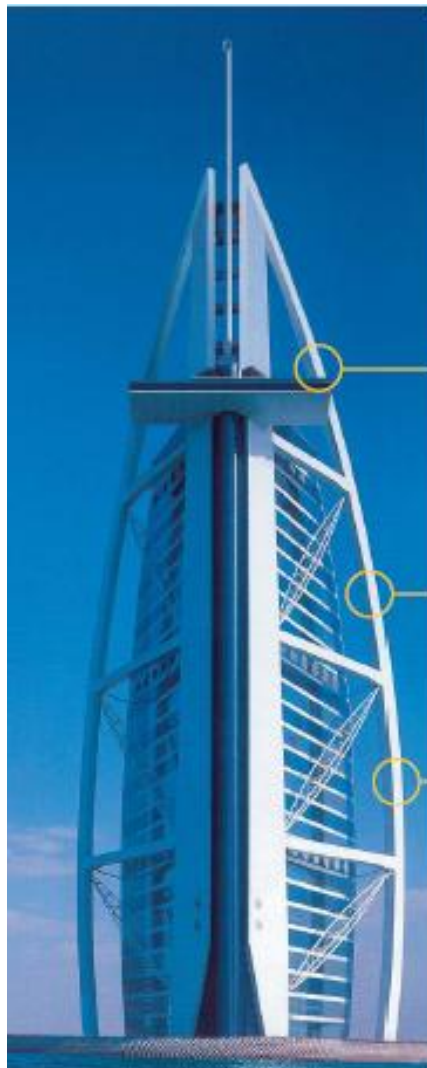
Figure 14. The Burj Al Arab contains a MTMD in its exoskeleton.
