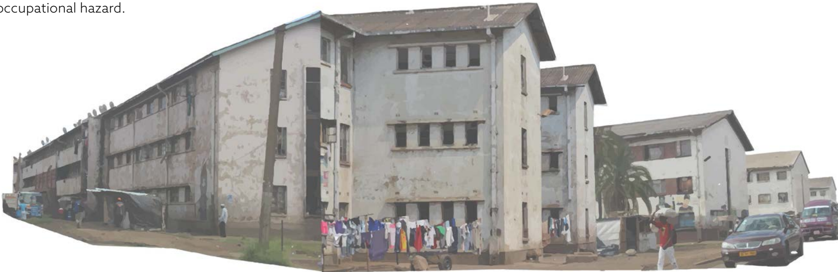
1_15. The state of hostels in Mbare now, overcrowded and structurally in poor condition.
