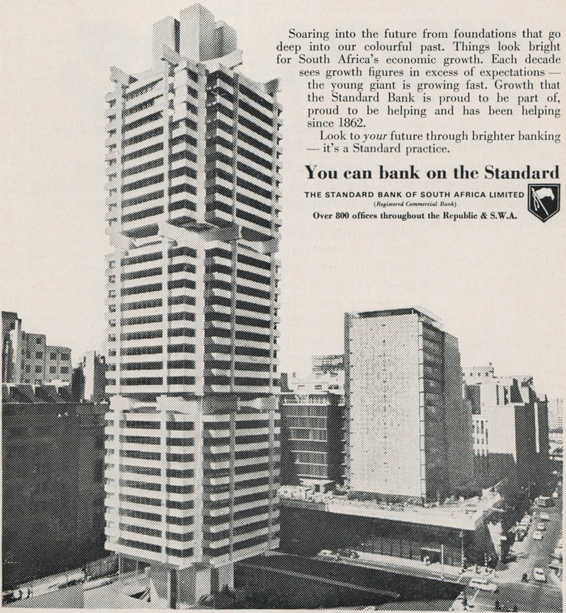
An architect's impression of the R16 million Standard Bank centre in Johannesburg.
