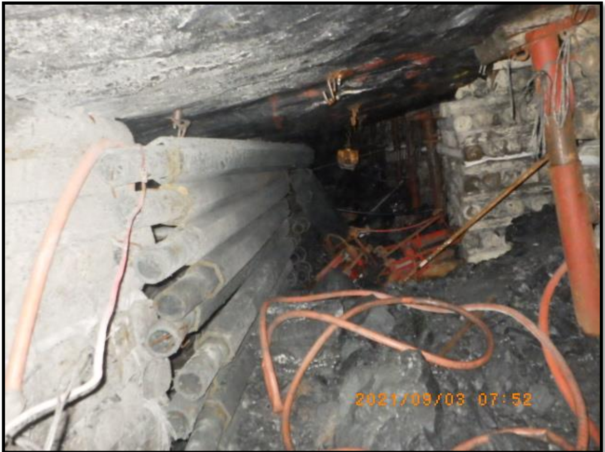
Figure 5-14: Ineffective installation of blasting barricades (Ndlovu, 2022)
