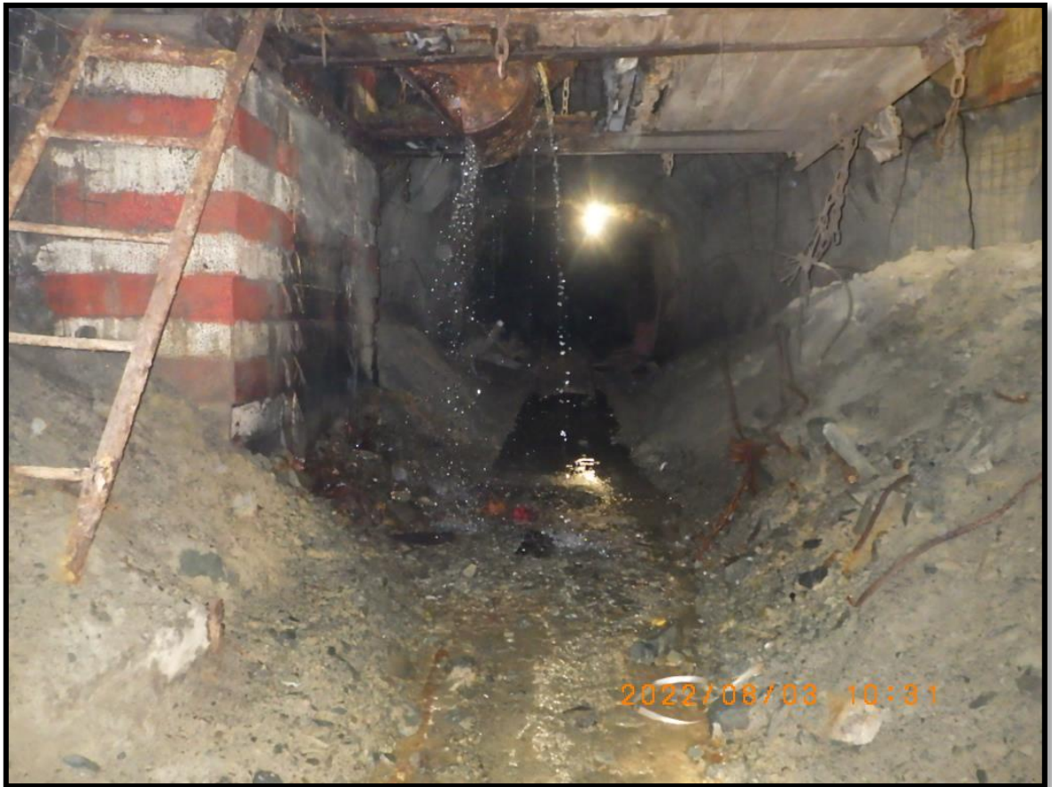
Figure 5-5: Accumulation of mud in the crosscut (Ndlovu, 2022)
