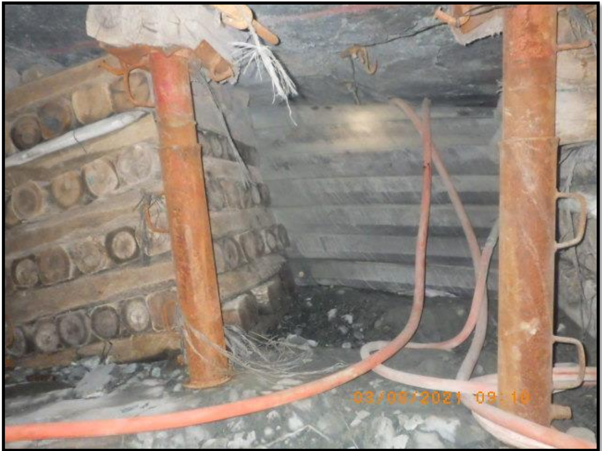
Figure 5-13: Effective blasting barricade installation (Ndlovu, 2022)
