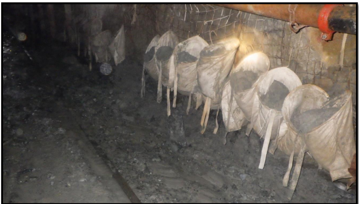
Figure 5-4: Mud bags hanging on the sidewall (Ndlovu, 2022)
