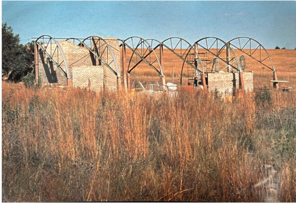
Figure 5:1 Under Construction (See Image credits)
