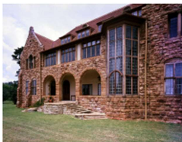
Northwards Herbert Baker Architect
