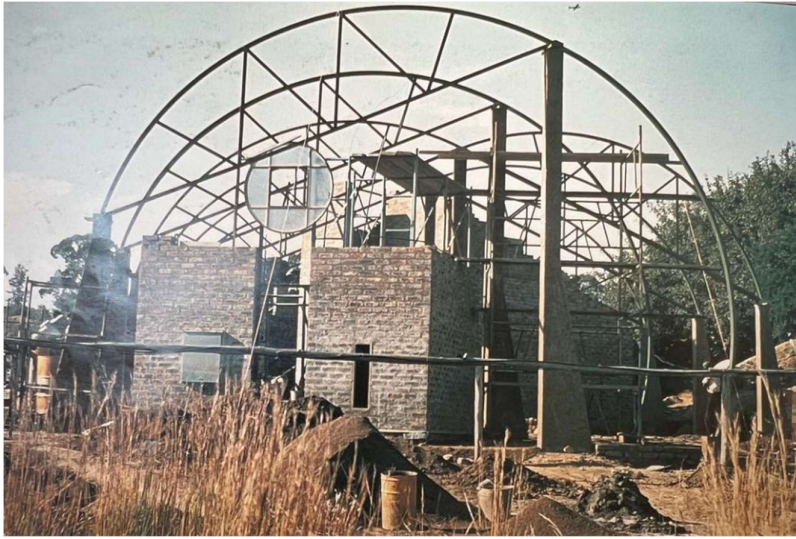
Figure 4:19 Under Construction (See Image credits)
