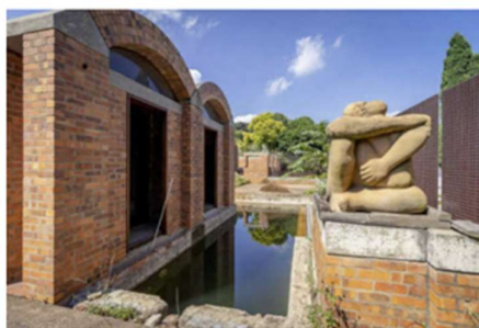
House Cohen, 1985 – Pancho Guedes Architect
