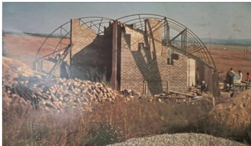
Figure 4:18 Under Construction (See Image credits)
