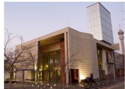
Constitutional Court, 1997 - Architects Urban Solutions and OMM Design Workshop
