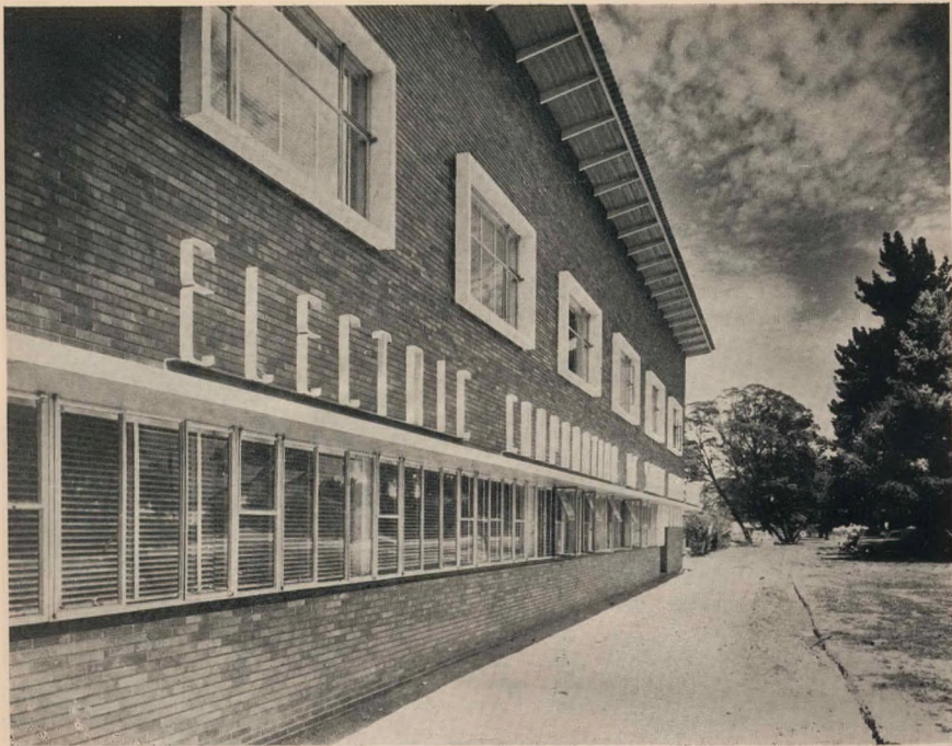
VIEW OF MAIN FACADE FROM ENTRANCE TERRACE
