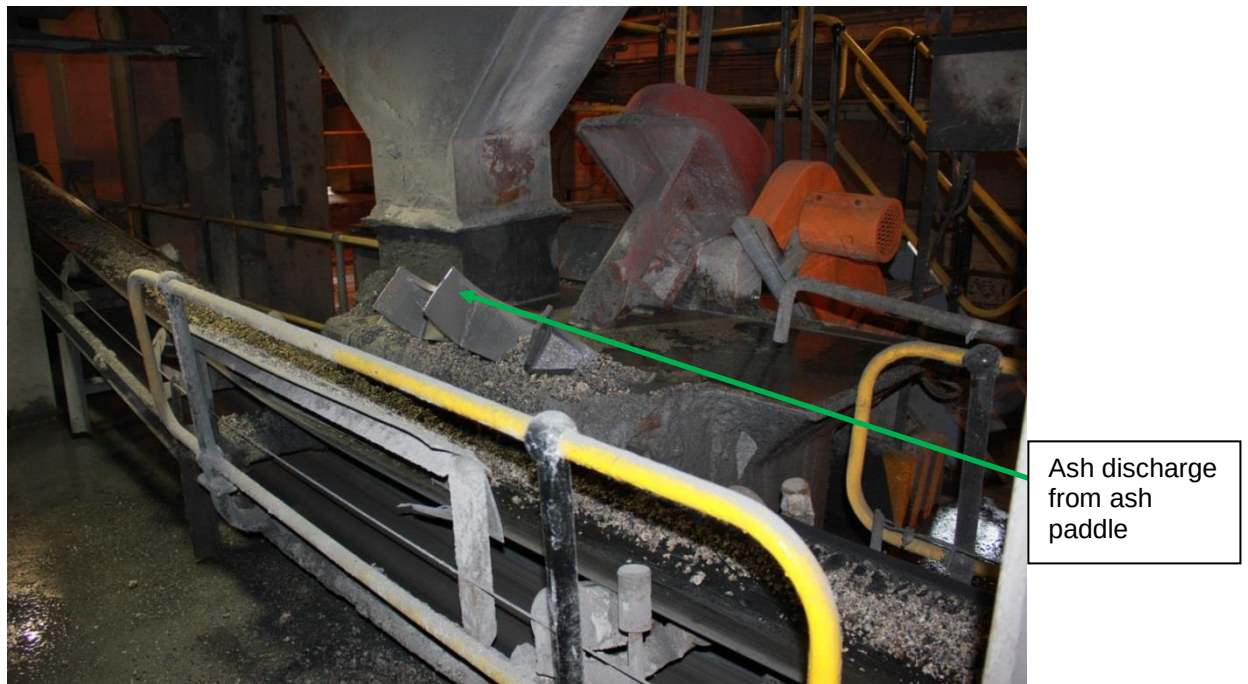
Figure H2: Bottom ash disposal System.
