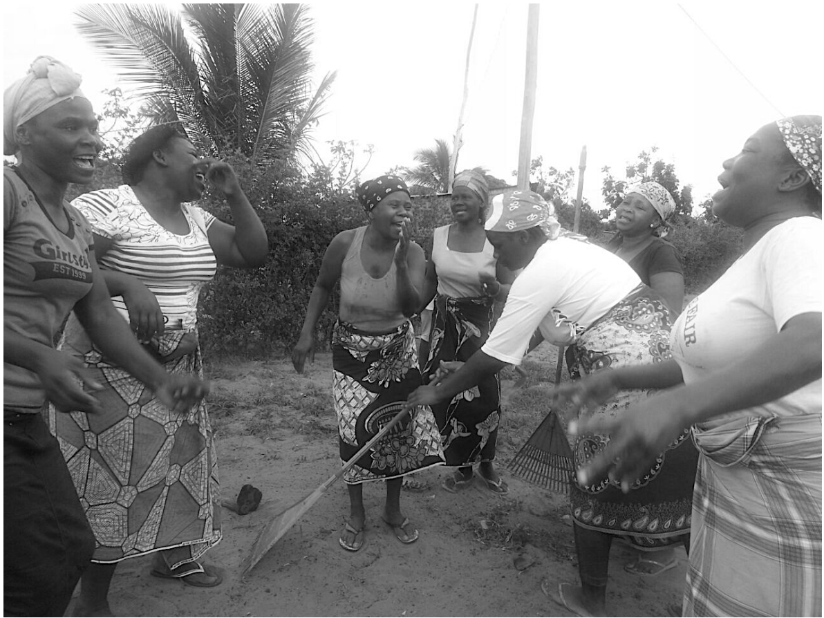
Figure 39: Picture of PASP workers clearing roads in Inhassoro, Inhassoro, 2017
