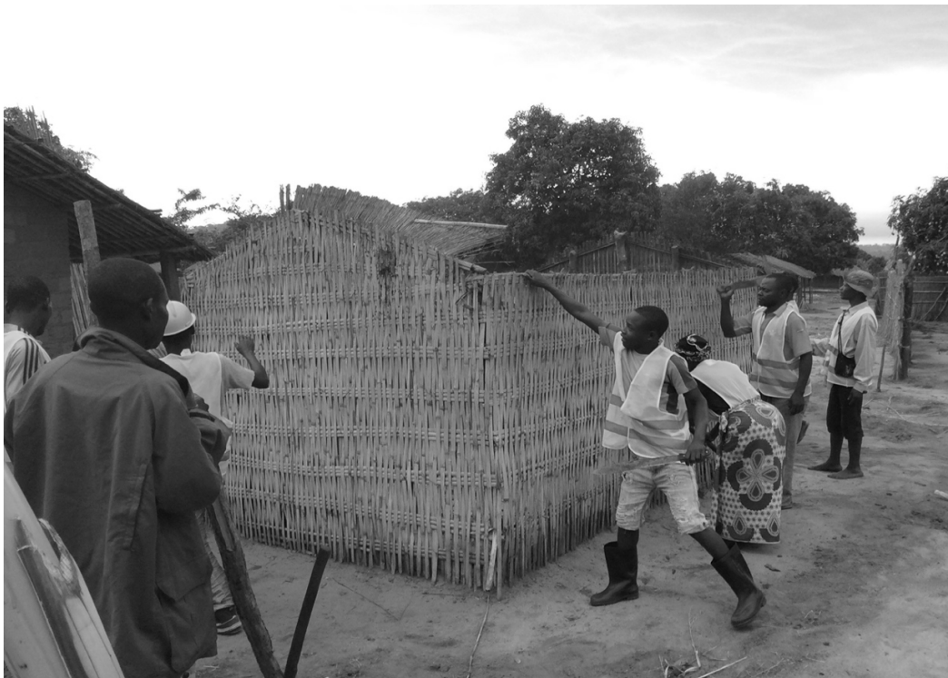
Figure 42: Picture of PASP workers demolishing a house in Riani, Ribáuè, 2017
