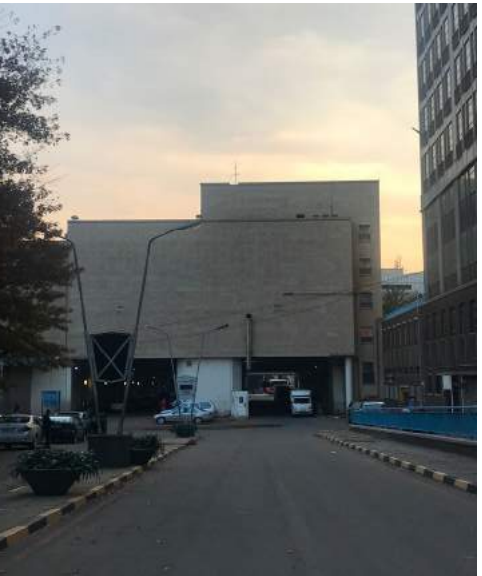
Figure 170: View looking at bridge
