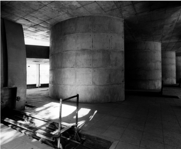
Figure 103: Fire chambers in Ashwinikumar crematorium
