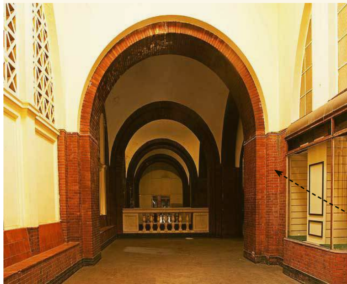
Figure 50: Old concourse building at Park Station
