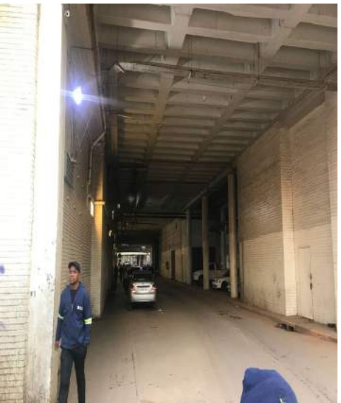
Figure 169: Approach from bridge
