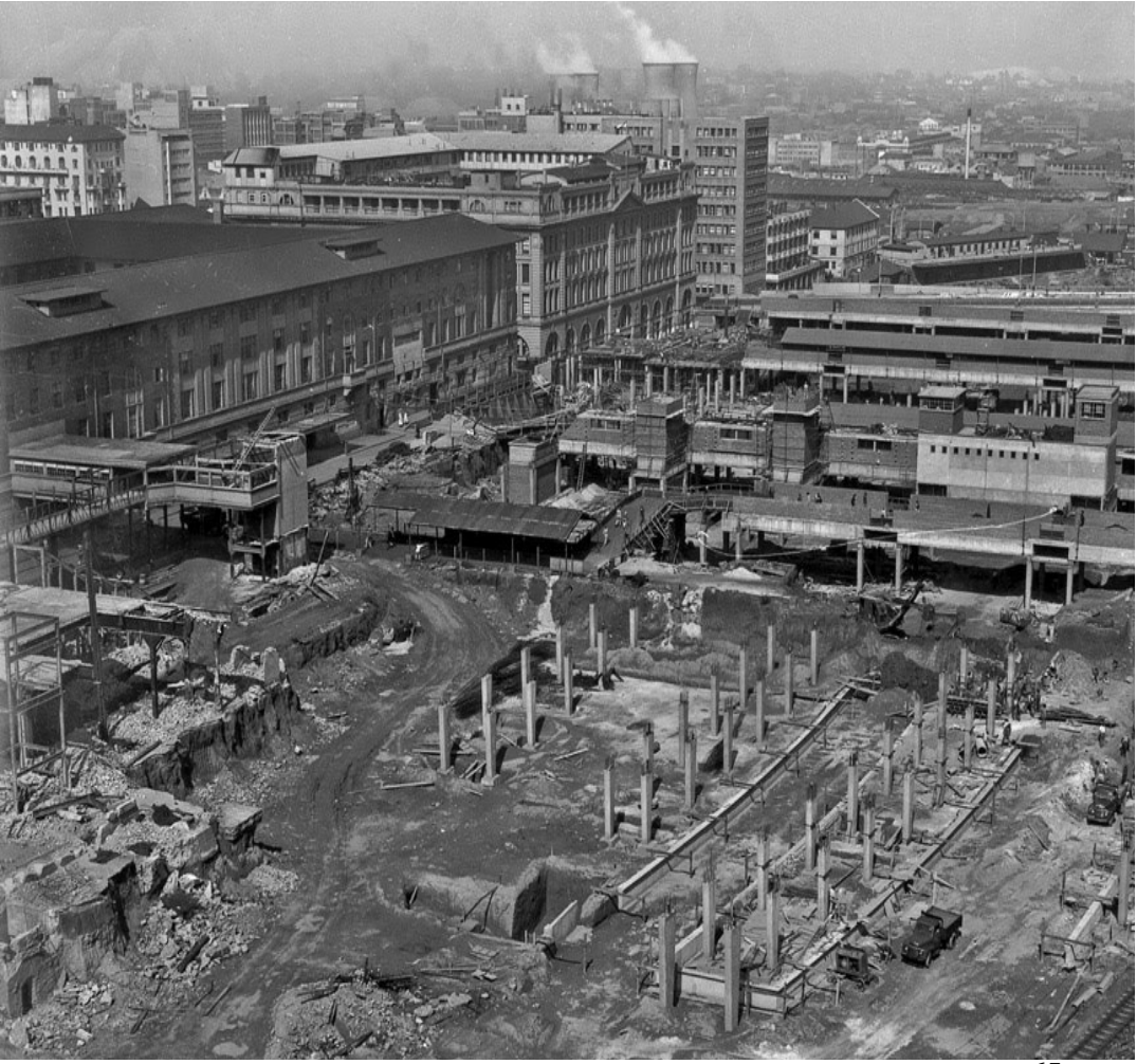
Figure 59: Park station under construction
