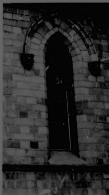
Window detail showing locally made brick and terracotta work by Church & McLauchlin.
