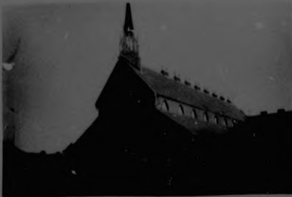
St Cyprians Anglican Church, a wood and iron building that was replaced in 1907 by the St Cyprians that we know today. The wood and iron churches such as this often tended to be a lot more Gothic than the brick buildings that followed. The church pictured above was in fact the second St Cyprians, the first which had mudbrick walls is referred to on Page 20. Photo Kimberley Public Library.
