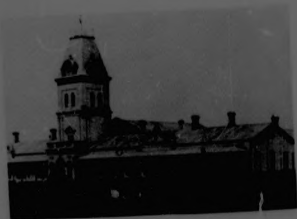
Worcester Free State Republic High Court Bloemfontein, built in 1877 as designed by Dutchman G. J. van der Merwe. It is a fine example of the building was afterwards, showing the resemblance to the original design.
