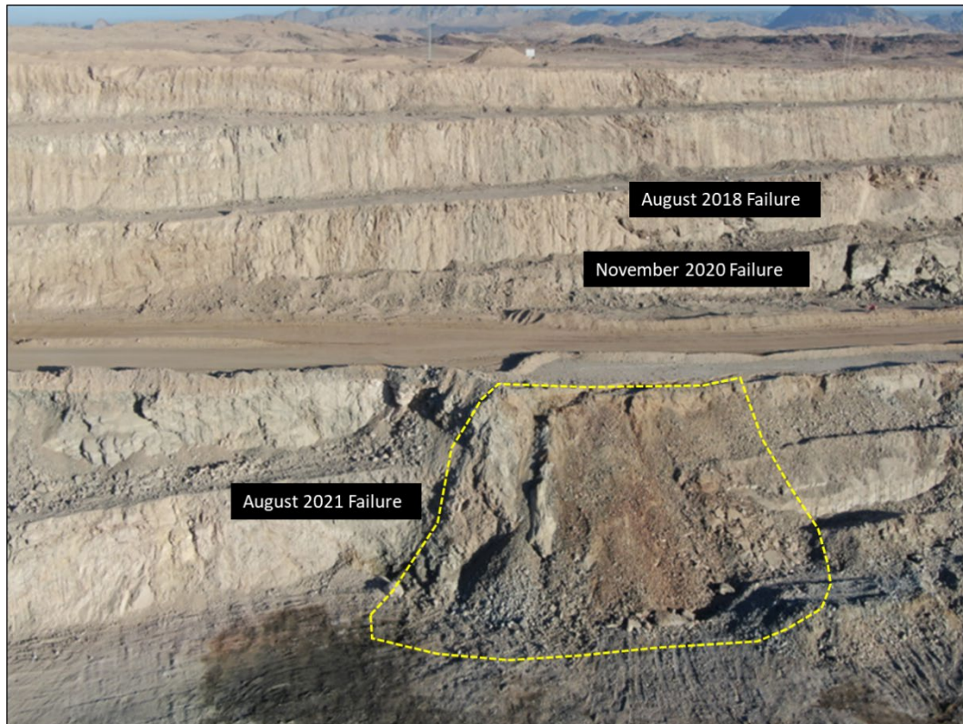
Figure 4-3: August 2021 failure taken with the DJI Mavic Air 2 Drone
