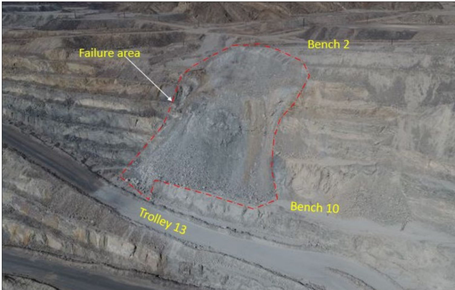
Figure 4-21: Failure in the Rössing Uranium Mine Open Pit – 31 July 2020
