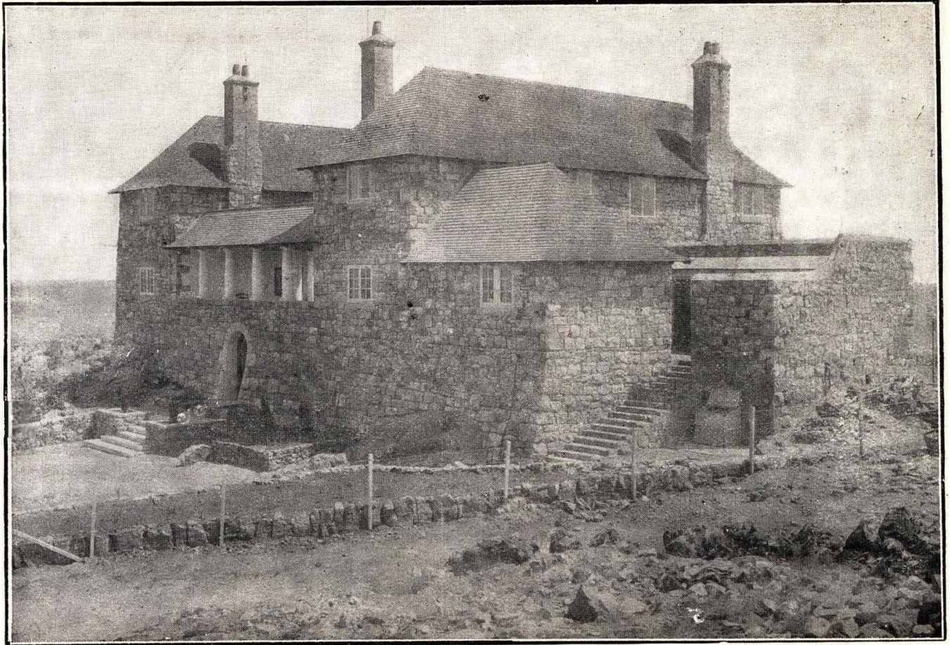
"STONEHOUSE," ETON ROAD, PARKTOWN FROM S.E. Residence of Herbert Baker, Esq., F.R.I.B.A.
