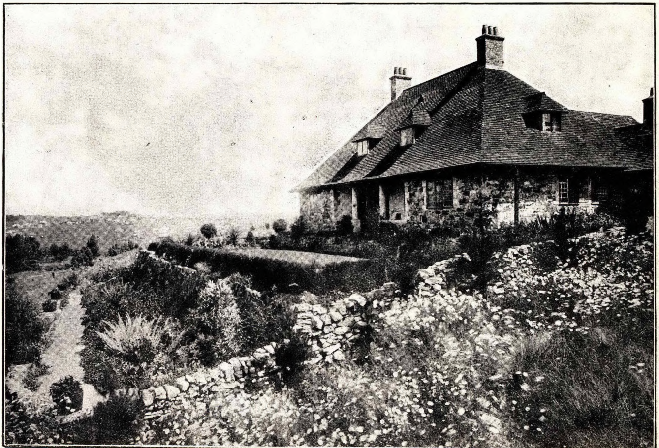
"ENDSTEAD," ESCOMBE AVENUE, PARKTOWN WEST, FROM S.E. Residence of the late E. Wilmott (E. W. Sloper).
