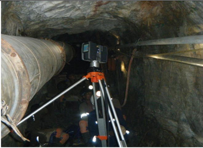
Figure 3.7: Faro laser scanner that was used to scan the actual shape of the material removed during the chipping process.
