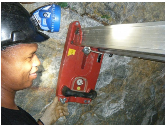
Figure 3.11: Securing the drill stand underground was much more difficult than anticipated.
