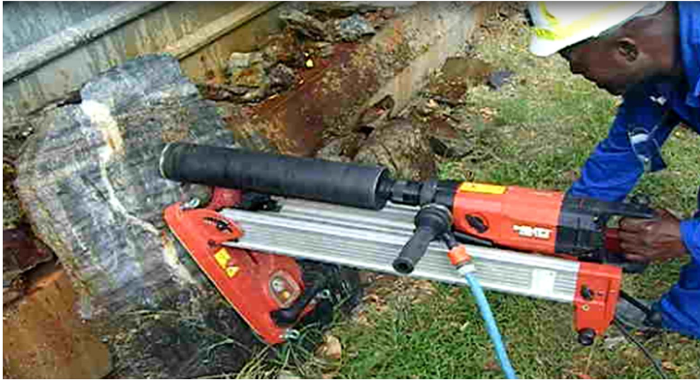
Figure 3.10: Drilling the core samples from a reef slab on surface was successful and promising.
