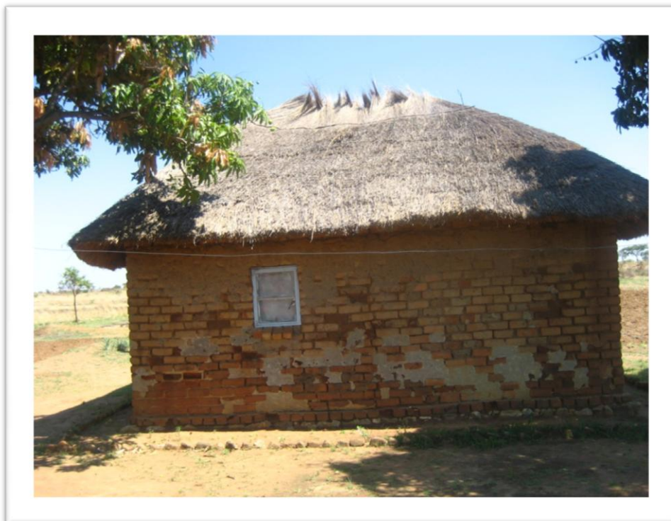
Picture 6.2: A kimberly brick and thatched house
