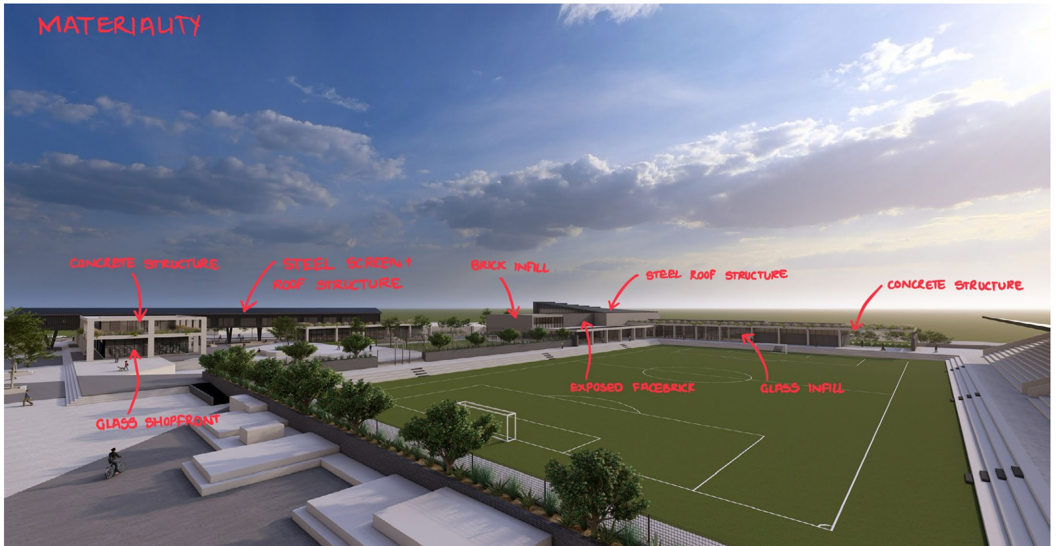
Figure 136: Building Materiality (M Rainho, 2024)
