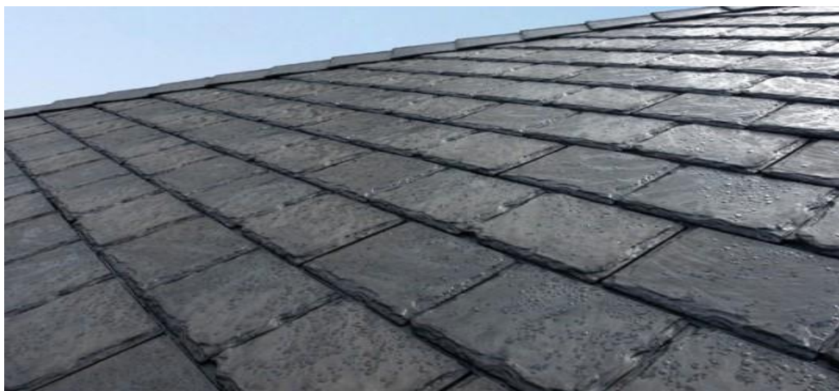
Figure 1.2. Roofing tiles made from waste tyres by Euroshield [28].
