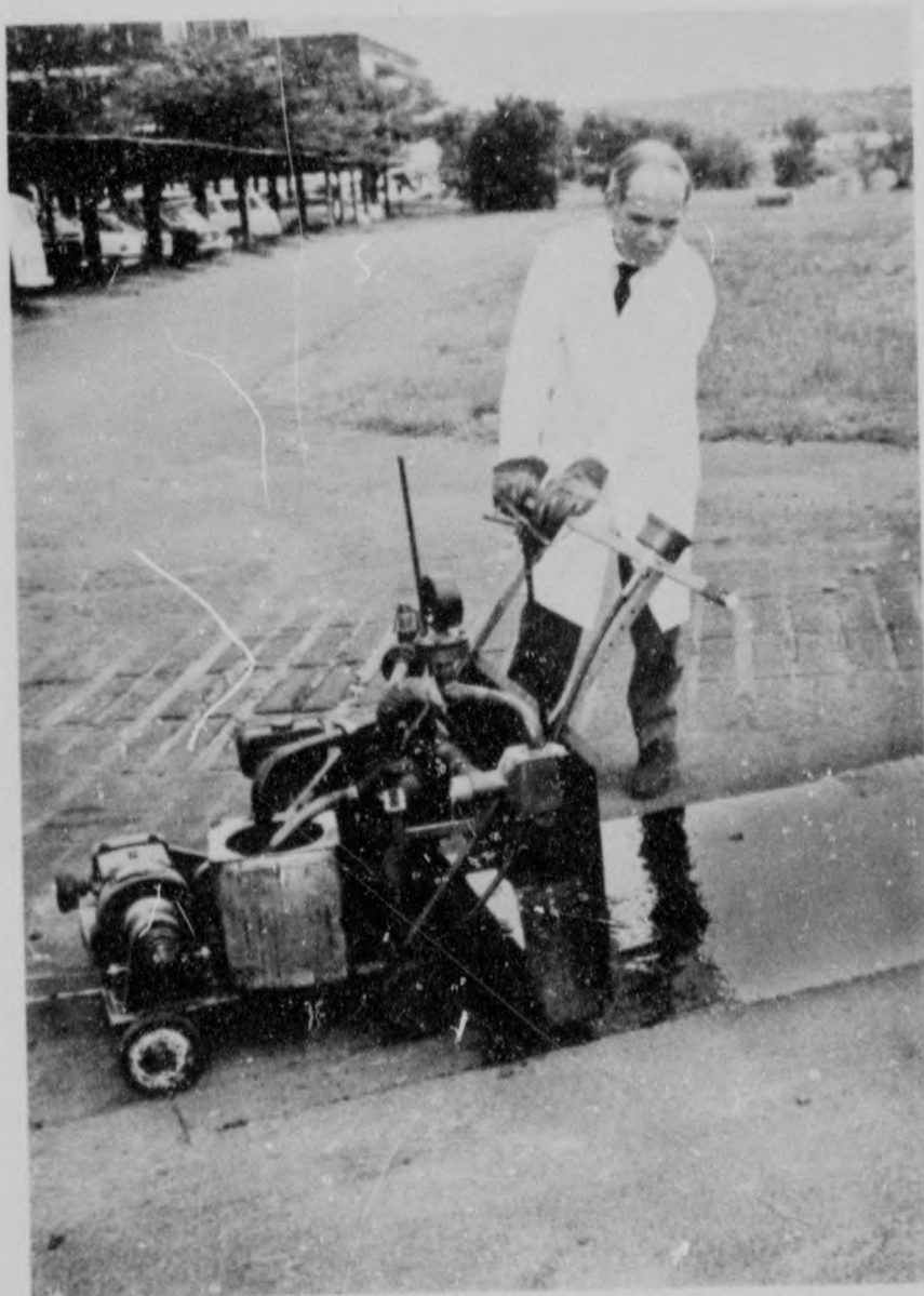
Figure 3 - 14: The mini binder distributor in operation.
