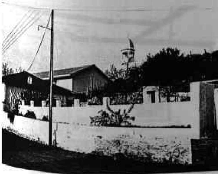
288. Erven 284 & 283: Wall of vacant lot, ? Bell Street.
