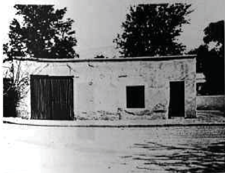
5. Erf ? (Old No. 0 1/2): Outbuilding, Bell Street.
