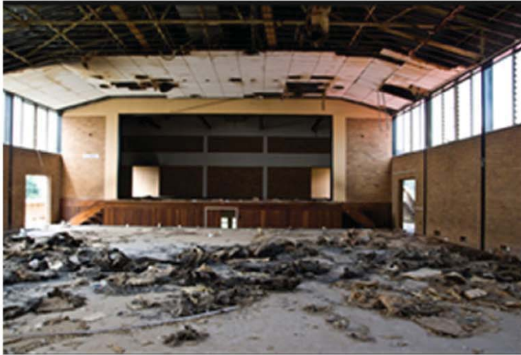
Figure 3.4: Photograph of Hall Space (1)_ Existing Primary School
