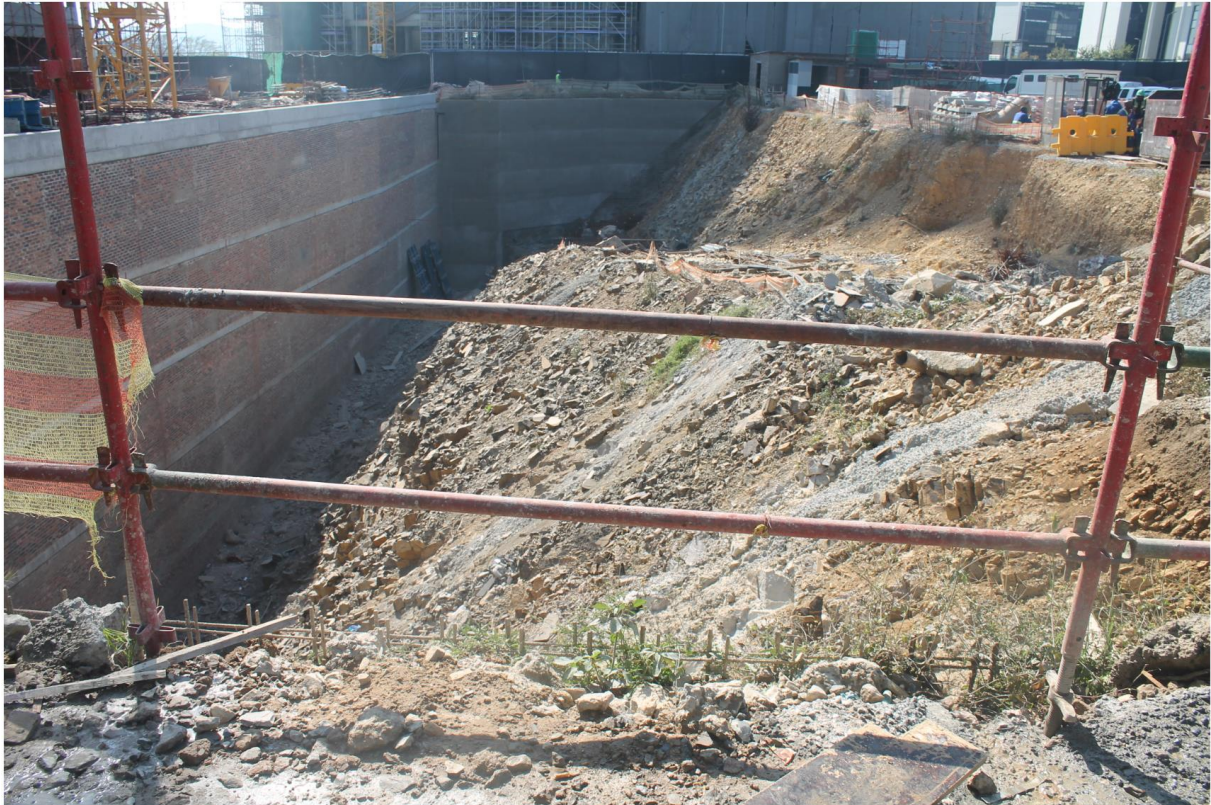
Figure 30: A view of trenches that will need backfilling with concrete and cement-based material.
