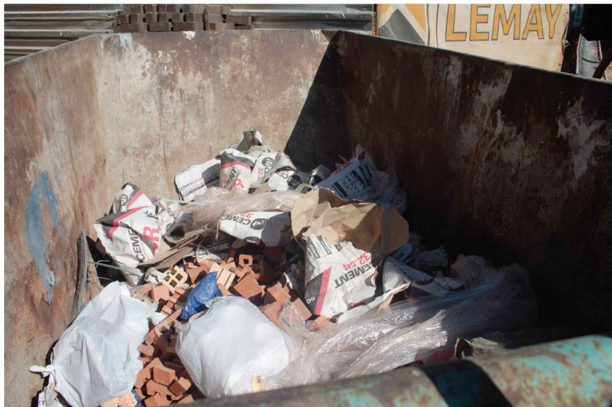
Figure 23: A view of the bin on site, which contained a mix of bricks, plastic and paper
