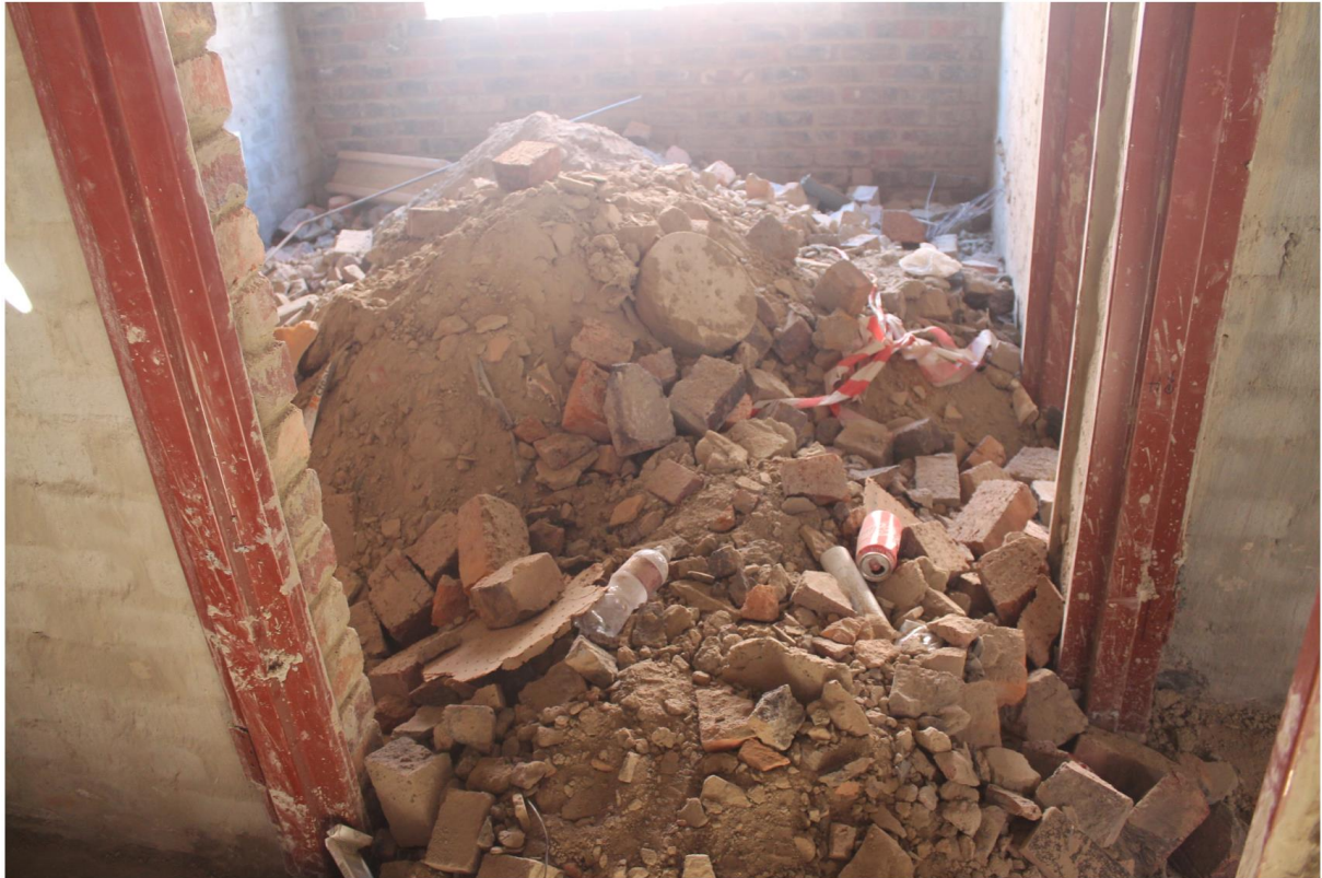
Figure 32: Waste concrete and bricks inside the building being constructed
