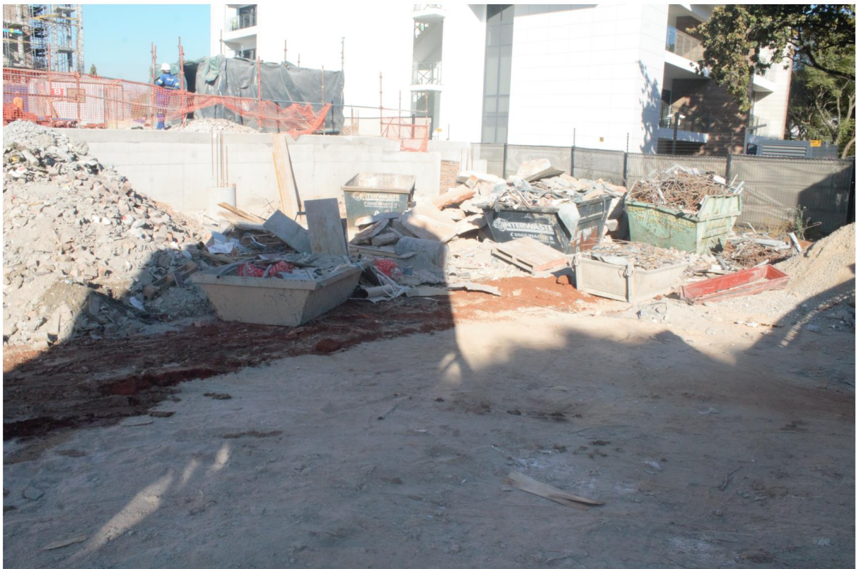
Figure 27: A view of the waste area which includes steel, plastic and paper
