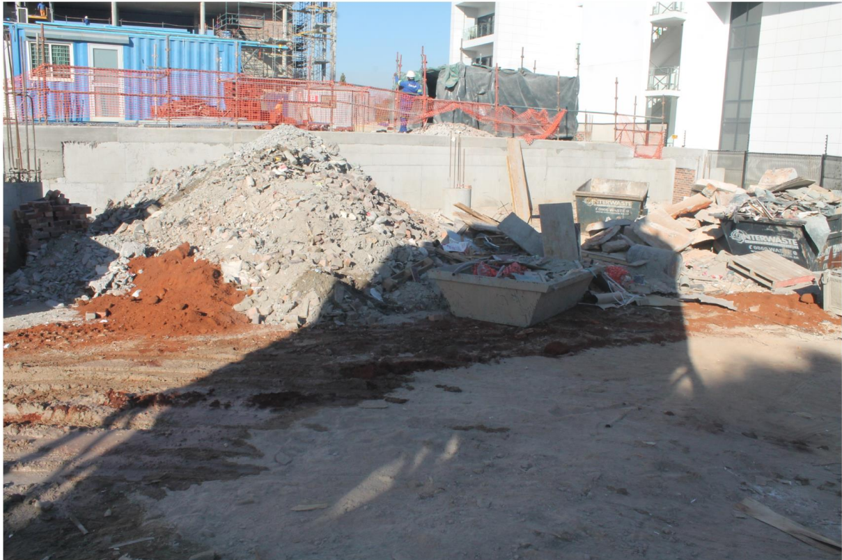
Figure 28: Waste concrete, bricks and soil to be used as backfill material
