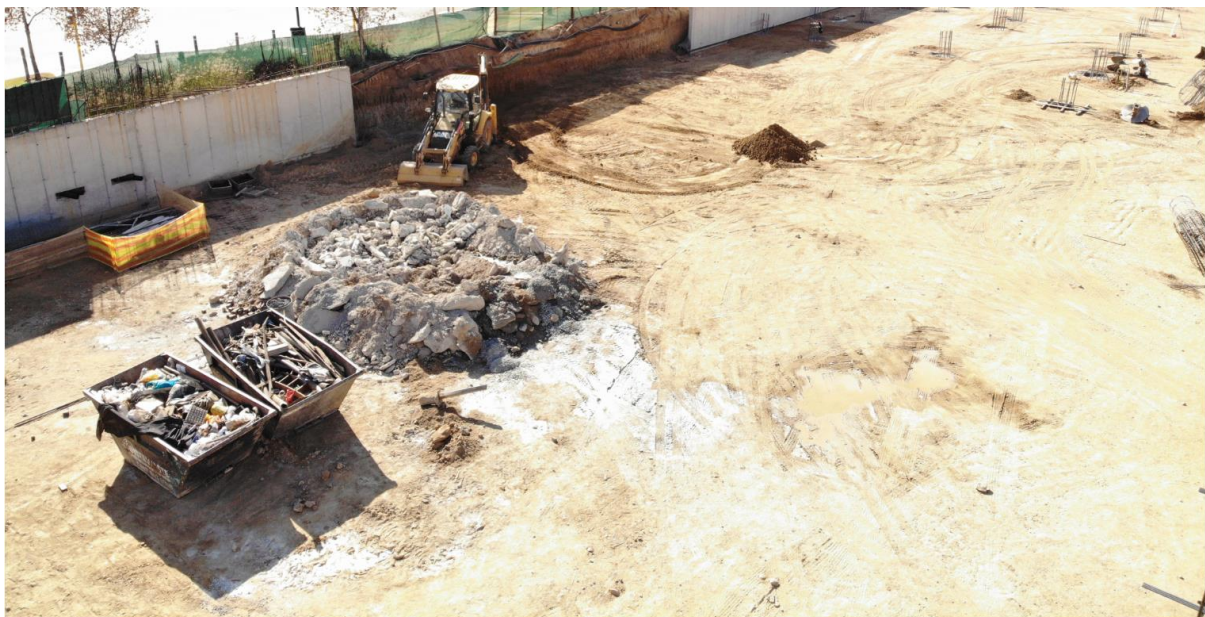
Figure 25: View of the bin area with waste steel, plastic and paper, and concrete sorted
