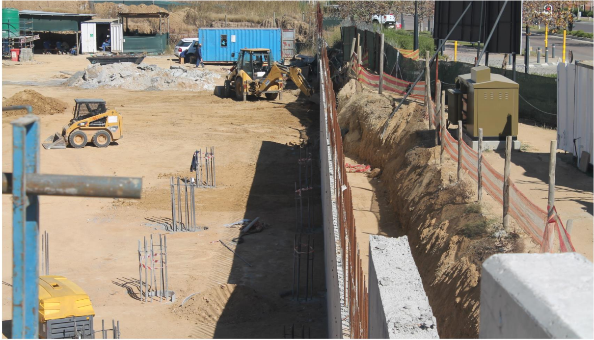
Figure 26: A view of areas trenches where waste concrete is used for backfill
