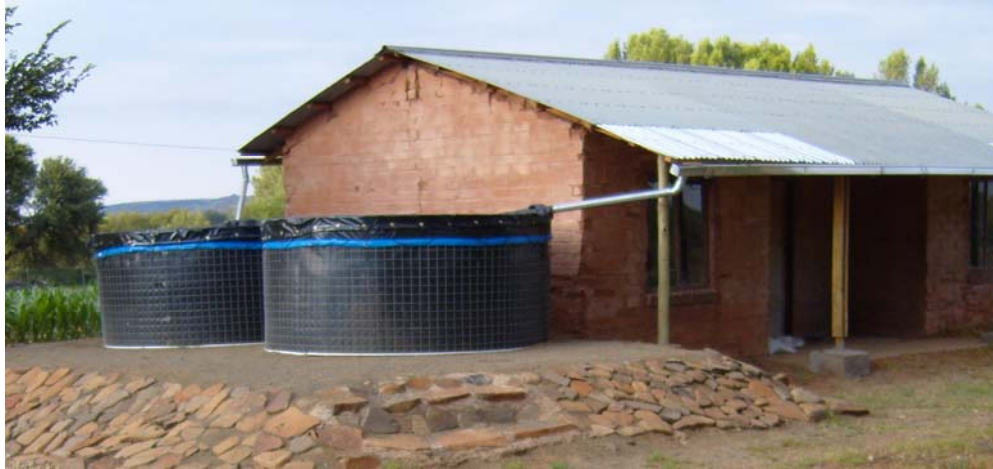
Figure 2.1. DRWH aboveground tank in Glen (Central South Africa).
