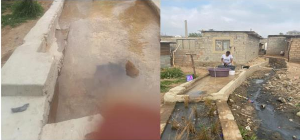
Blockage at side wetland
