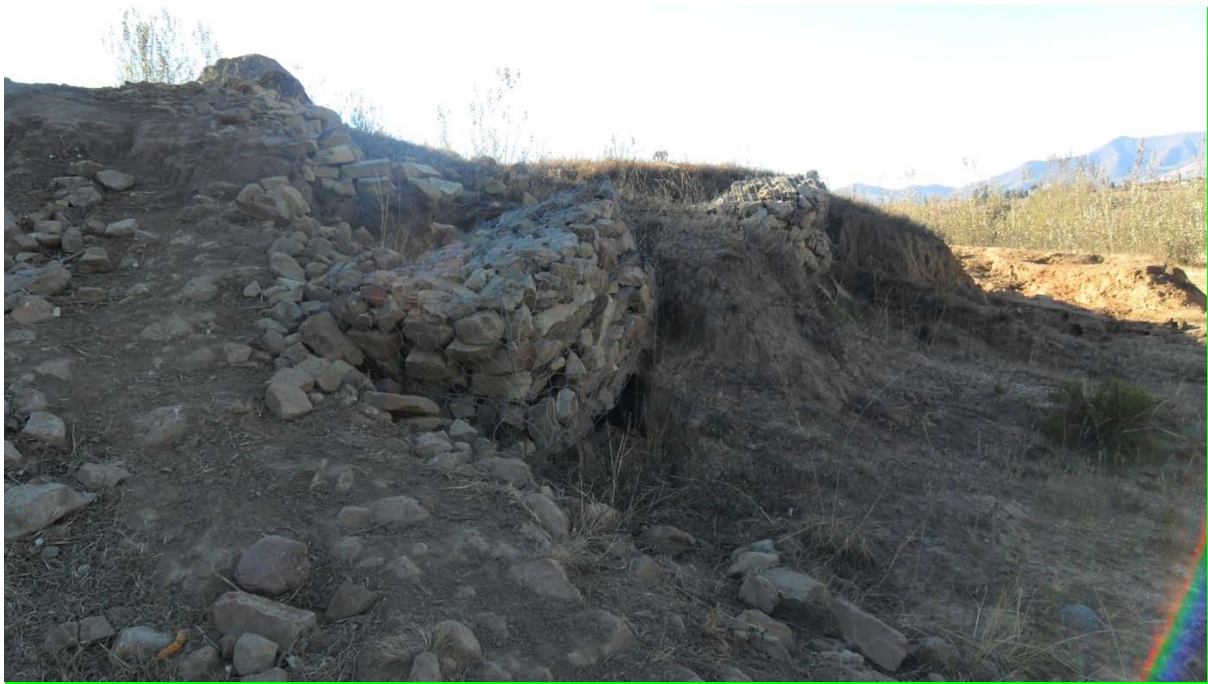
Gabions constructed as part of road rehabilitation during the Nursery Project tenure
