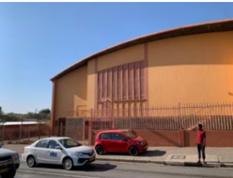
Figure 15: Katutura Town Hall 2024 (Author, 2024)
