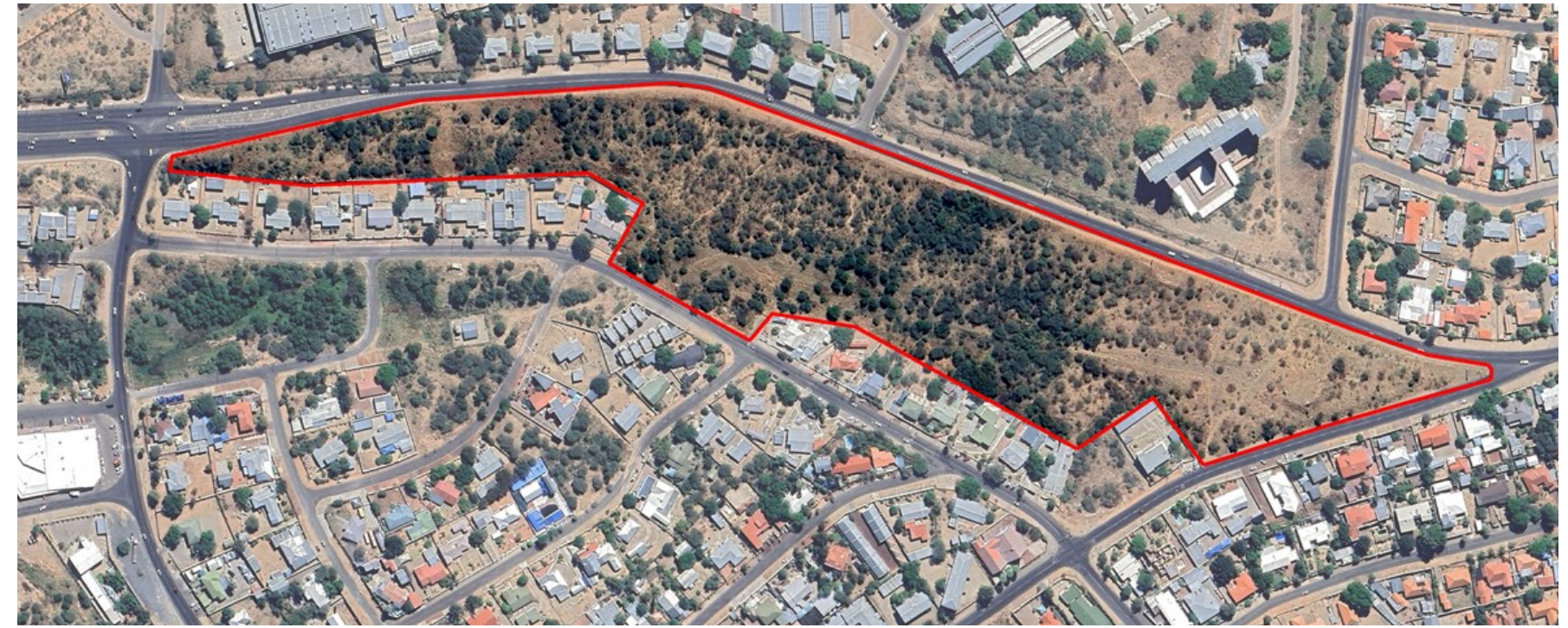
Figure 70: Site Aerial Photograph (Author,2024)
