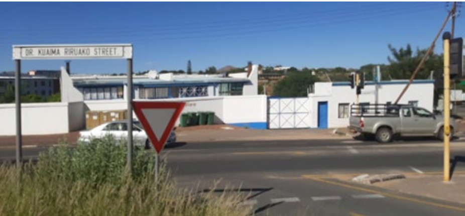
Figure 56: Roads of Windhoek West (Haindongo, 2024)
