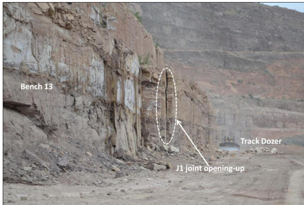
Figure 2.2: Orapa Mine pit inspection. Source: Orapa Geotechnical Engineering Department.
