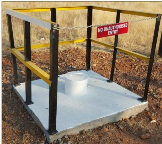
Figure 2.7: Benchmark photograph. Source: Orapa Survey Department.
