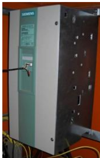
Figure 5.2: Siemens Simoreg DC master digital converter/drive
