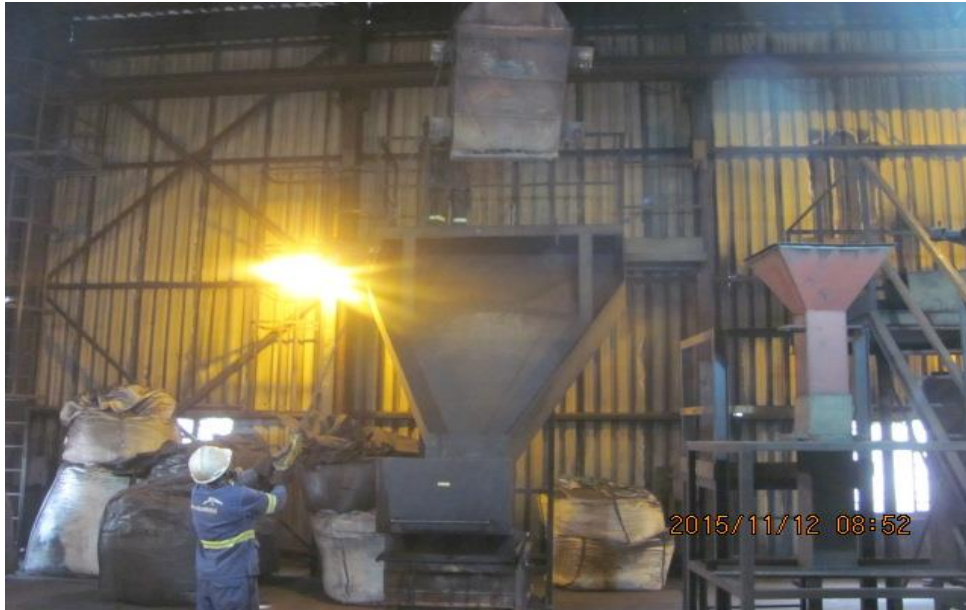
Figure 11: Stabilisation of the coke by use of the stabilising chute
