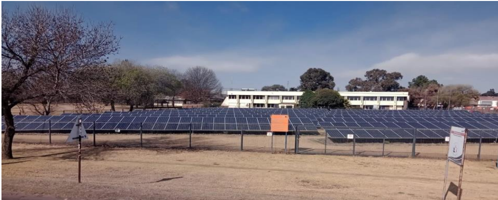
Figure 14: Solar panels on arable land in Mpumalanga
