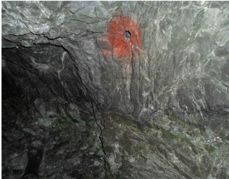
Figure 44, Poor face profile and advance resulting from a pull-out/misfire in the fifth Emulsion B blast.
