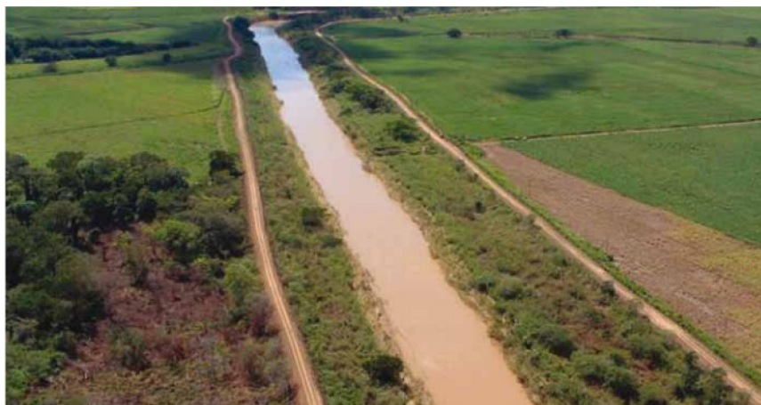
Figure 3.5: The canalisation of the Mfolozi river was constructed to reduce flooding, but it led to an increase in water velocity and suspended sediment (photograph: Ezemvelo KZN Wildlife).
