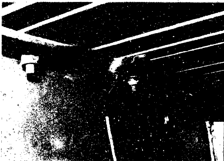
Photograph 5.73 Two core electrical supply cable clipped to underside of deck next to side rail
