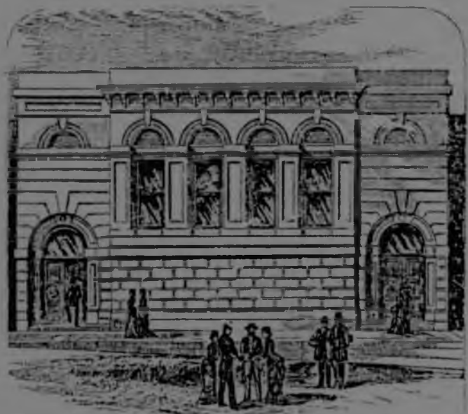
BAPTIST CHURCH W, WALE STREET. 1862 C. FREEMAN (BAPTIST CHURCH)
