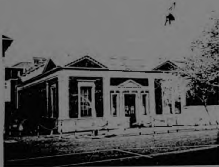
S.A.C. PHYSICS BUILDING,
