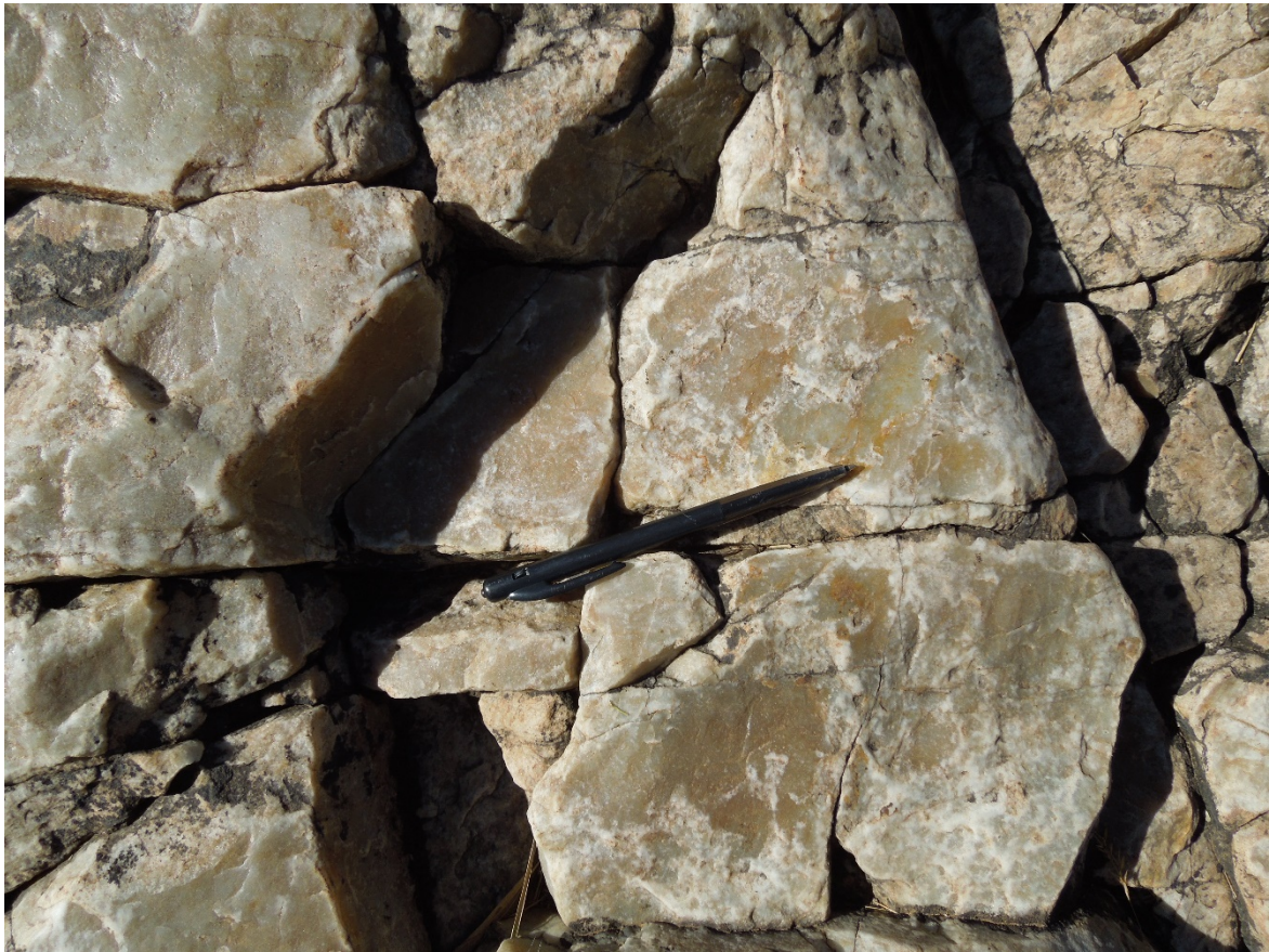
Figure 2.22: Highly fractured quartzite in the Vredefort Dome (*pen shown for scale) Courtesy of Mr Khuliso Masindi).
