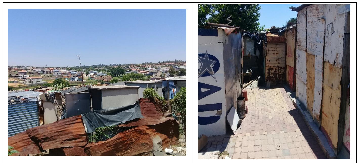
Figure 4.2 Photos of clustered and connected (linked together) shacks in Msawawa and Kya Sands, a possible fire hazard. Source: Author's own photo 24 th September, 2017.
