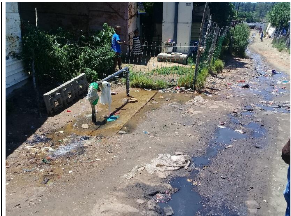
Figure 4.11: A photo of leaking stand water pipe in Msawawa
