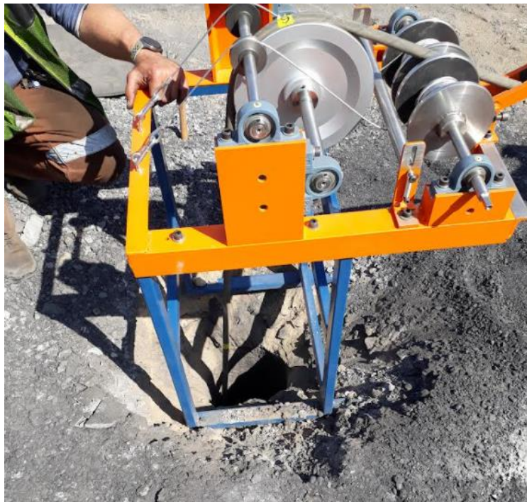
Figure 3.1 : Hot-hole with spraying machine
