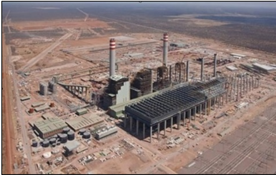
Figure 2: Medupi Power Station under construction (Lephalale Municipality, 2013b)
