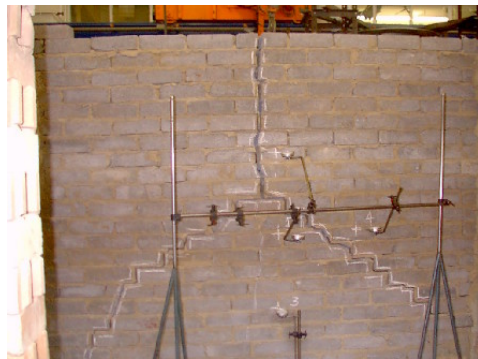
Figure 4.11 Mode of failure standard conventional masonry (medium span)
