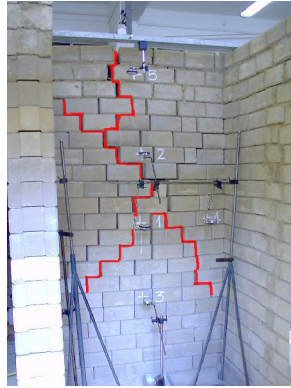
Figure 4.5 Mode of failure short span wall
