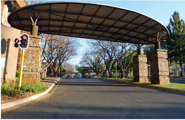
FIGURE 32: Entrance to secure office park near Wanderers, Colette Drive
