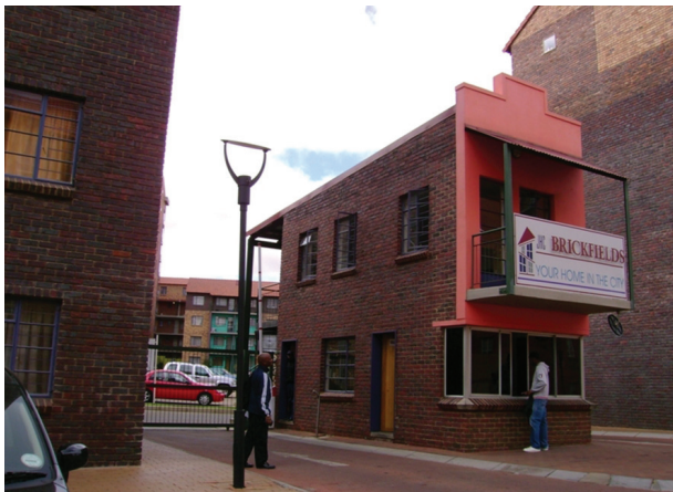
FIGURE 30: Entrance gate and guardhouse to a large mixed-income housing complex in the inner city of Johannesburg. Access is controlled through gates and security guards with CCTV surveillance cameras.
