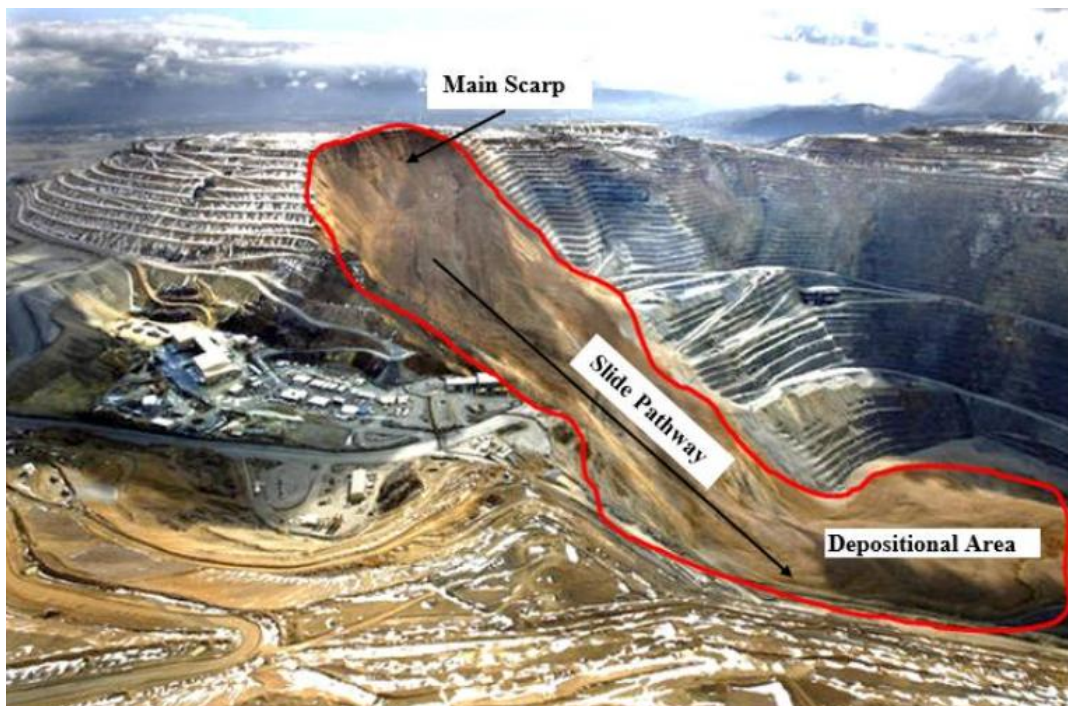
Figure 26 - Slope failure at Kennecott Utah Copper's Bingham Canyon mine (Kolapo et al., 2022)
