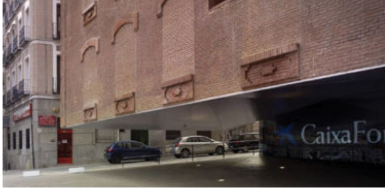
Fig 7.18 The Caixa Forum, Herzog and de Meuron Architects, 2008 entrance detail (Image @ Christian Richters, www.arcspace.com/architects )
