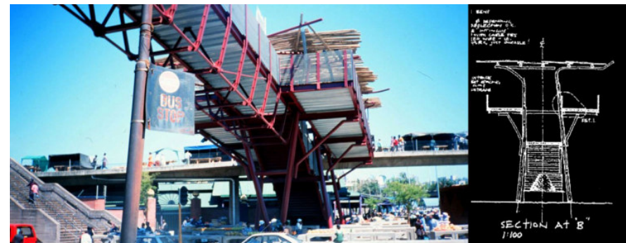
Fig 7.31 Warwick Junction market precinct, OMM Design Workshop market road bridge roof detail (Courtesy OMM Design Workshop)
