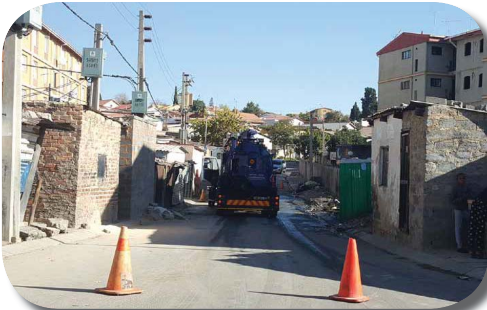
Figure 4.2. 08 : Insufficient bulk services. Alexandra, Johannesburg.
