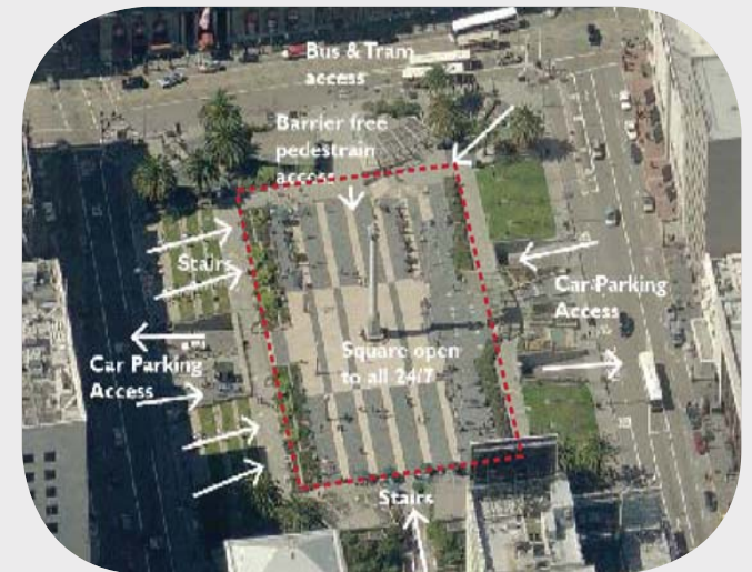
Figure 5.1.06 : Union Square Aerial View
