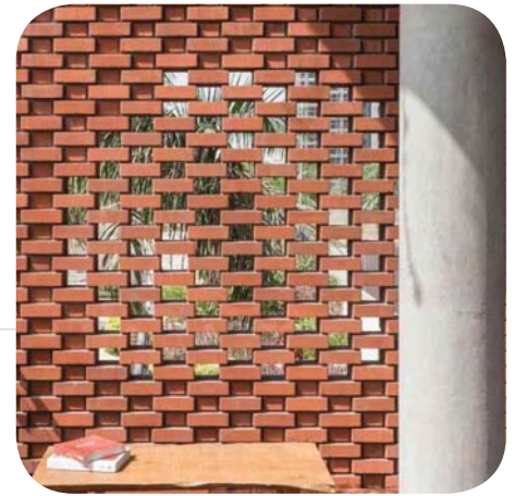
Perforated brick and round column
