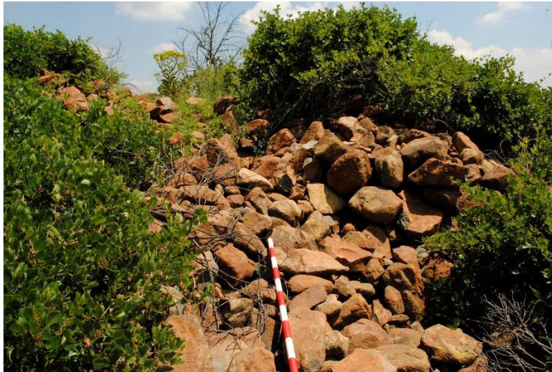
Photograph of Raised Structure 52
