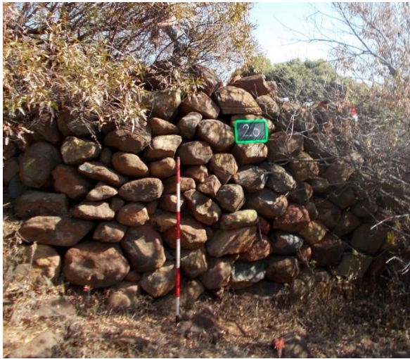
Photograph of Raised Structure 26
