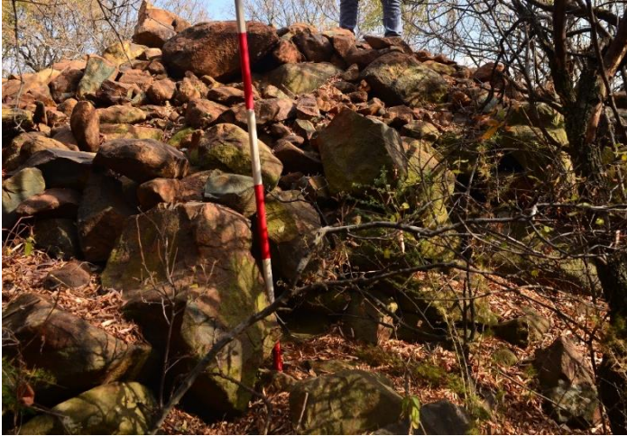
Photograph of Raised Structure 5 (meter stick for scale)
