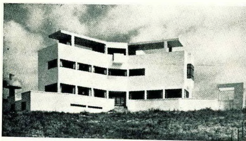
HOUSE AT AMERSHAM 1932
