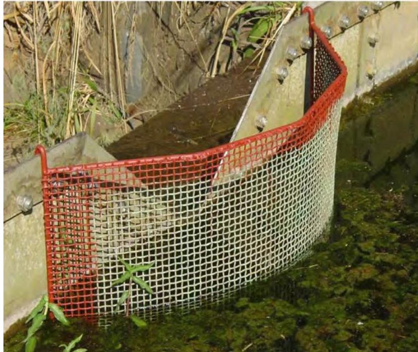
Figure 4.14: The V-notch weir located along the river of the Two Streams larger sub-catchments (Everson et al. , 2014).
