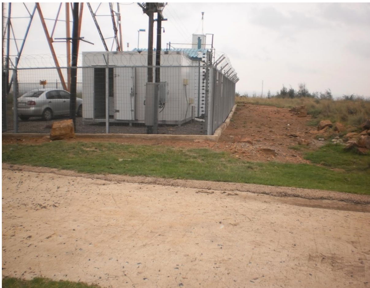
Figure 4: Photo of Elandsfontein monitoring station showing the surrounding grassland
